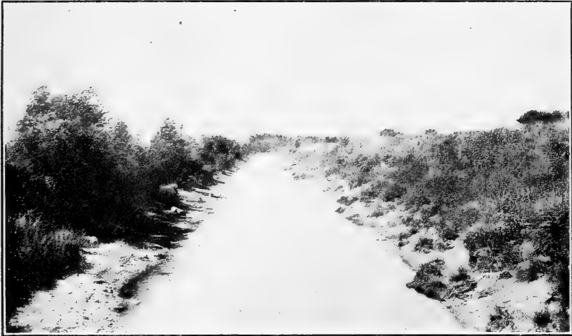
FIG. 1.—SLOPE COURSE OF LITTLE SIOUX RIVER CUT-OFF DREDGED CHANNEL, NEAR TURIN, IOWA, 1916. (SEE TABLE NO. 4.)
